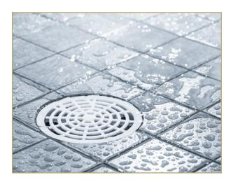
Install trap primed drains in floor drains and other applications that may see infrequent water use (for example, guest shower drain, basement floor drain). This will help prevent sewer gas from finding its way into the house.
